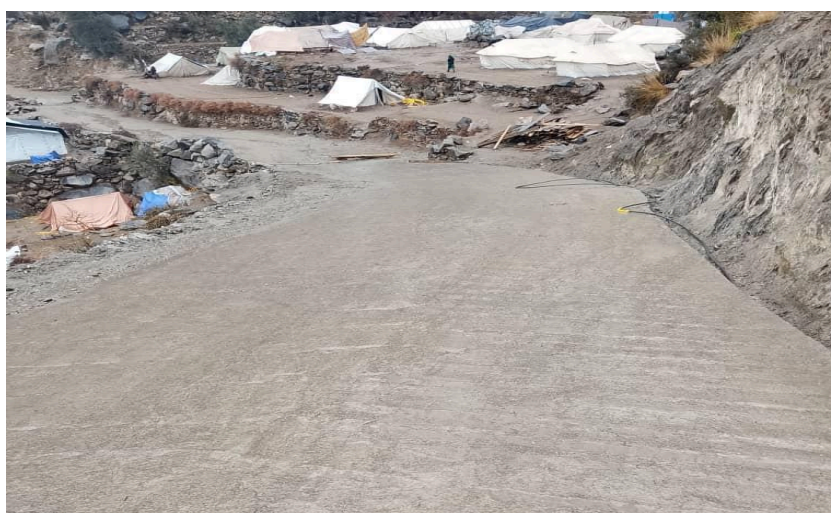
Rehabilitation of Ander Lachak Road under the Earthquake Response in Kunar District complete December 2025 @FP/DACAAR
