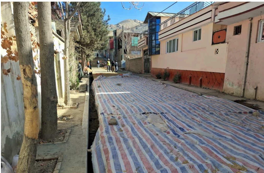
Implementation of cold weather measures at a plum concrete street in Gozar #19, District #17, Kabul City, December 2025 @UNOPS
