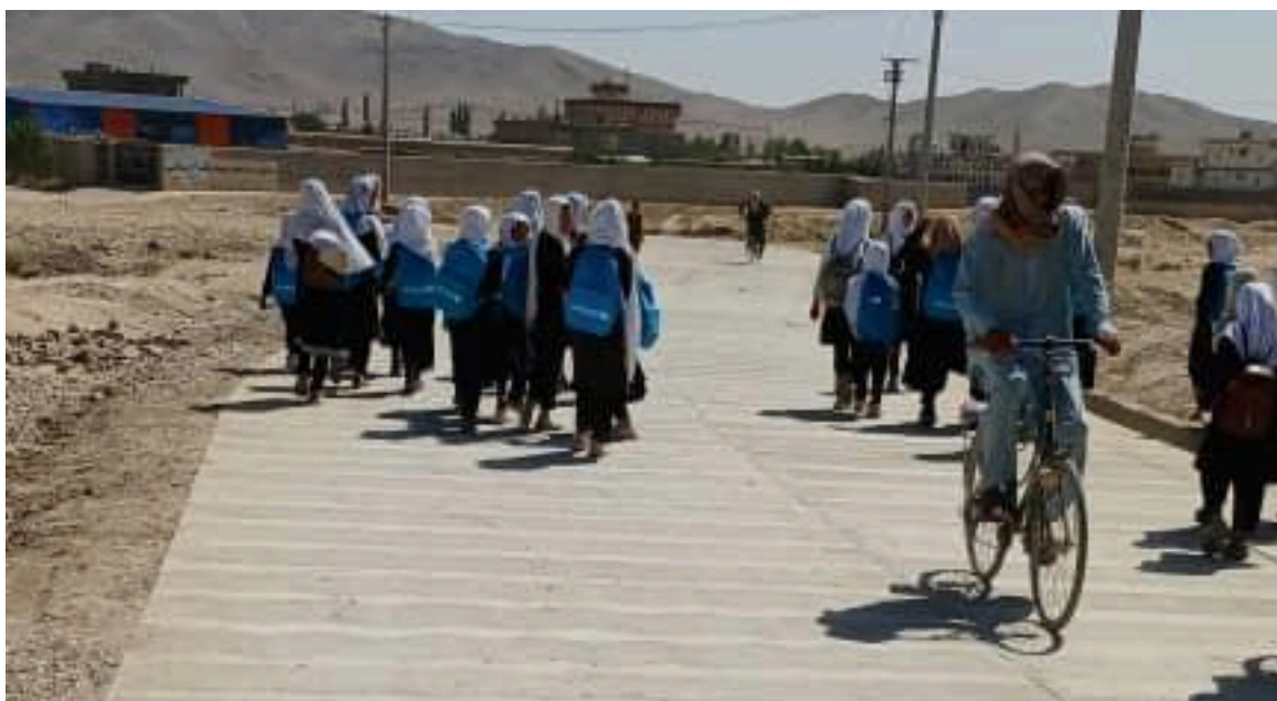
School children from a nearby girls' school are benefiting from improved access through the Arbaba to Qala Ashrat street paved with Plum Concrete surface(L=505m), Gozar#2, District#4, Ghazni City, 17 September 2025 @UNOPS
