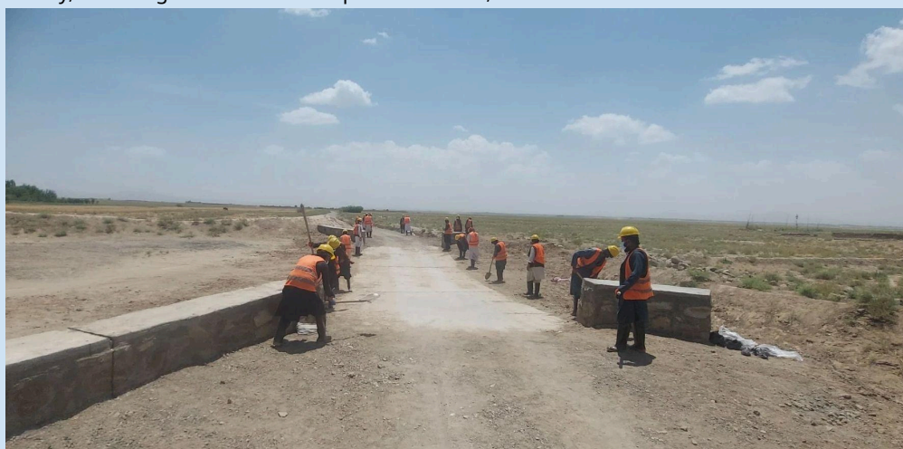
Ahmad Khan working along other laborers on road rehabilitation @FP CDDO
