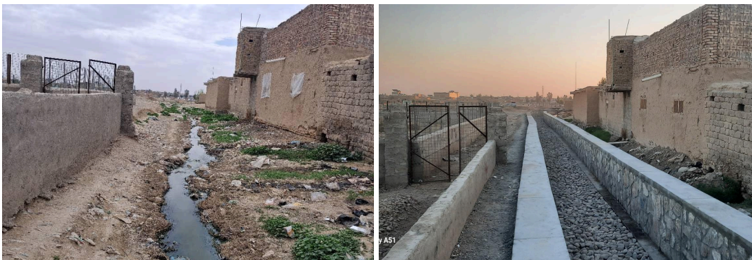
Before and after photos of a surface water and flood control canal in Gozar #1, District #14, Kandahar City on 25 Nov 2025 @UNOPS
