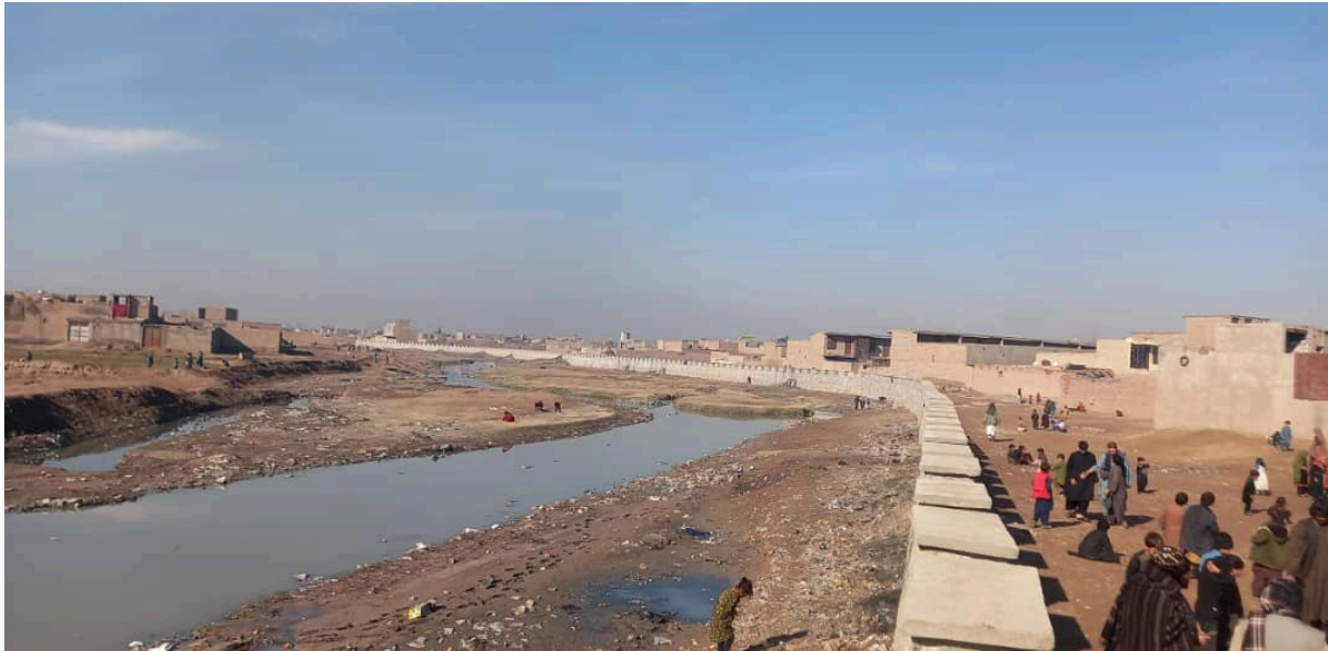
Flood protection wall completed in Gozar 6 District #10, Herat City in September 2025 providing a shield for homes, people and livelihoods @UNOPS
